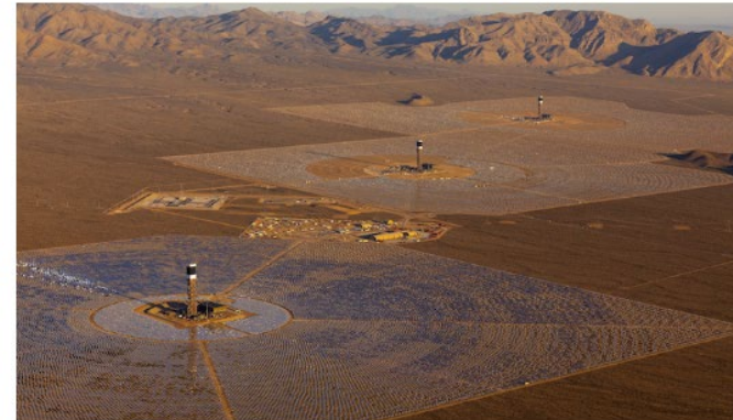
General Plant Data
