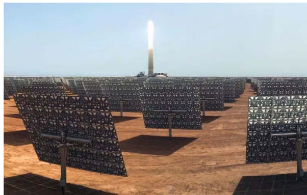
Fig. 2 Sener's HE54 heliostats at Morocco's Noor III facility (operational since 2018). At 178.5 \text{ m}^2 , this is the largest heliostat in commercial CSP use [1]. Each facet uses a latticed support. This reduces the material usage of the facet itself, a weight reduction which can lower design loads on the drives and heliostat structure. Adapted from Ref. [67].
