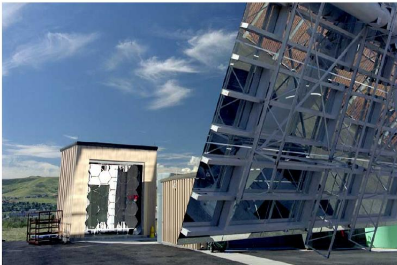
At the top of NREL's South Table Mountain campus, the HFSF is a unique user facility for testing high-
