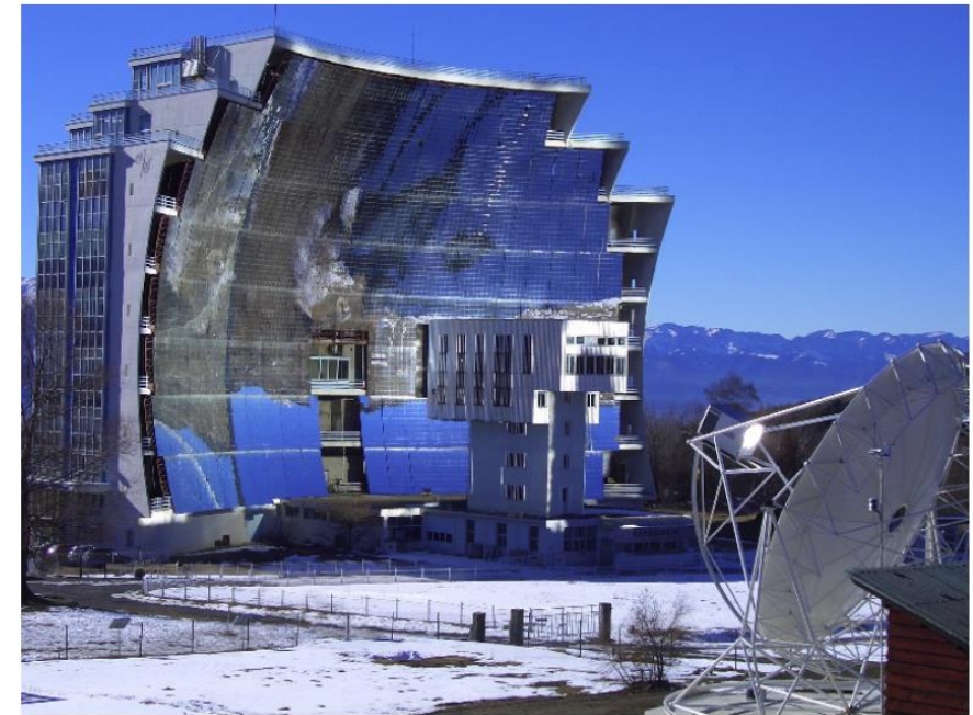
Figure 1.4. Solar furnace of CNRS at Odeillo-Font-Romeu. In the foreground, the dish-Stirling module being tested
