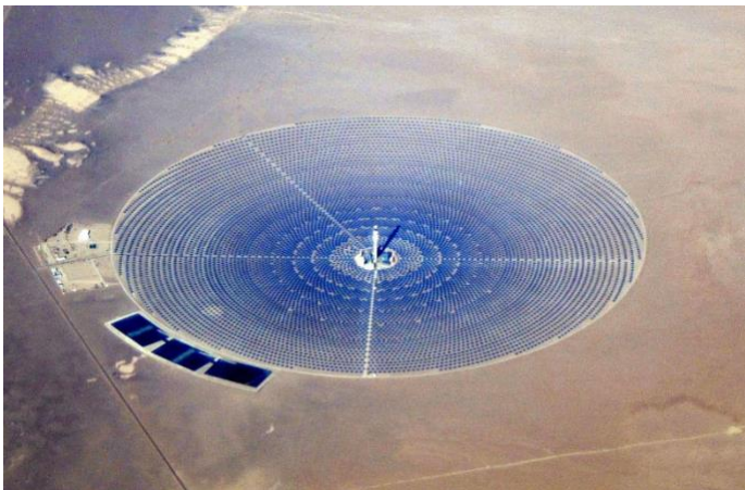
Figure 5: Crescent Dunes power tower plant, aerial view [b]
