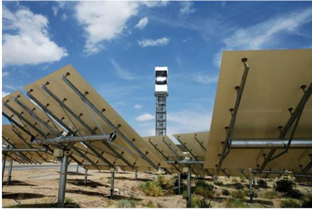
Figure 13: T-bar heliostat support with pins [f]
