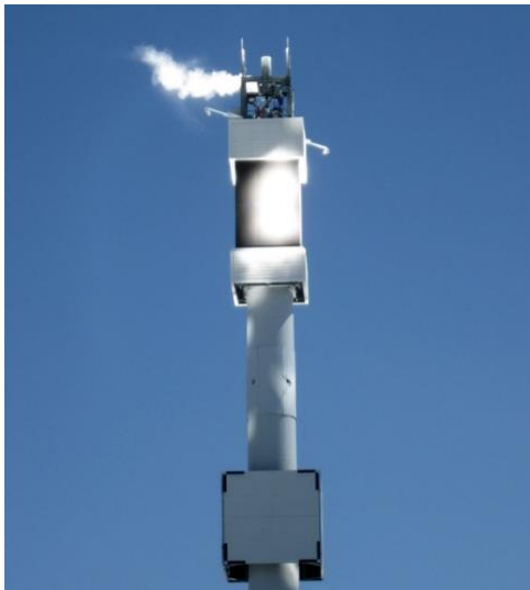
Figure 21: External Receiver at Sierra Suntower in Lancaster, CA
