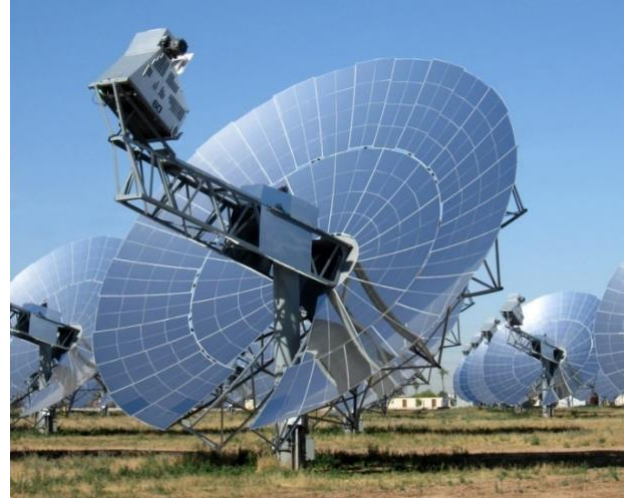
Figure 4: SunCatcher 38-ft parabolic dish collectors
