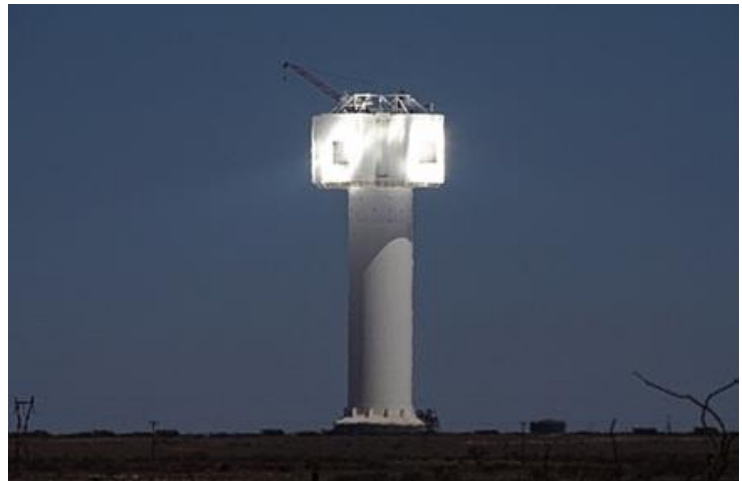
Figure 22: Cavity Receiver (with spillage) at Khi Solar One [n]
