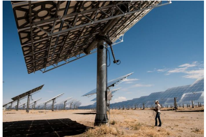
Figure 12: Scale of heliostats, stamped backing
