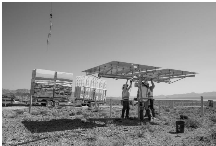
Figure 25: Heliostat installation at Solar Field One in 2012 [q]
