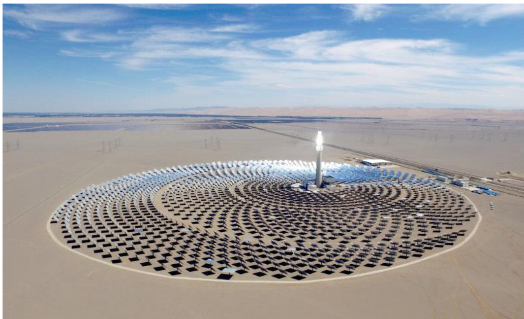
Figure 24: Radial Heliostat Field at Shouhang Dunhuang [p]
